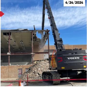
• 4/24/2024 The high reach backhoe made its maiden voyage and began removing the roof structure of the natatorium.
