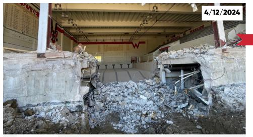
• 4/12/2024 Peitzmeier removed the concrete structure between the blue gym and the Natatorium to create a ramp down into the empty pool. The pool slab was cut and removed along with the deep end pool walls and deck.
