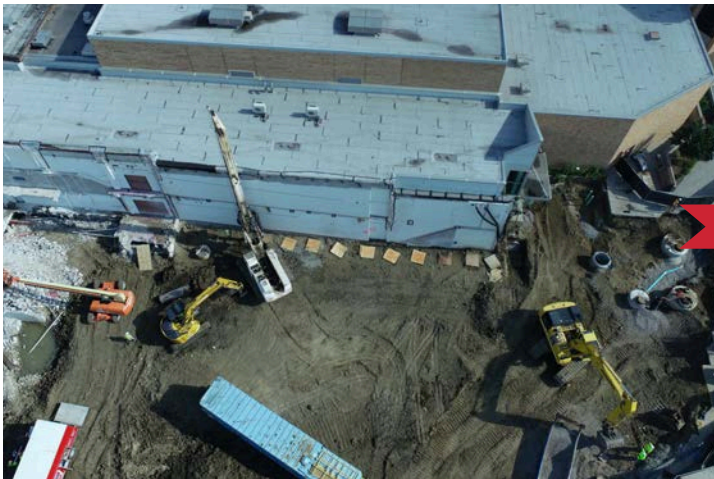
• 6/13/2024 Drilling of soldier piles for soil retention.
