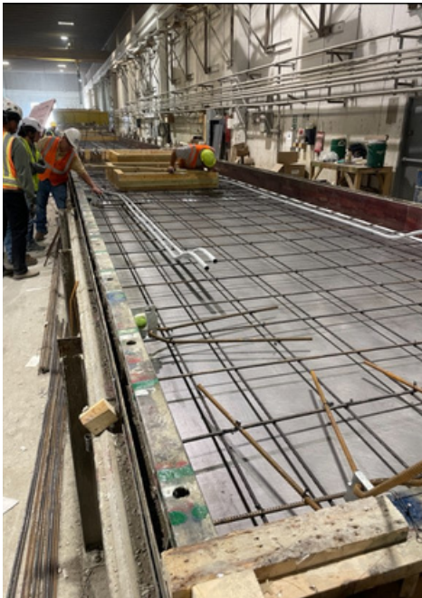
10/2/2024 Precast Panel Fabrication at Coreslab. All panels are cast and currently being 'groomed' to their final finish. The precast panels will makeup the south and west exterior walls and the west wall of the natatorium.
